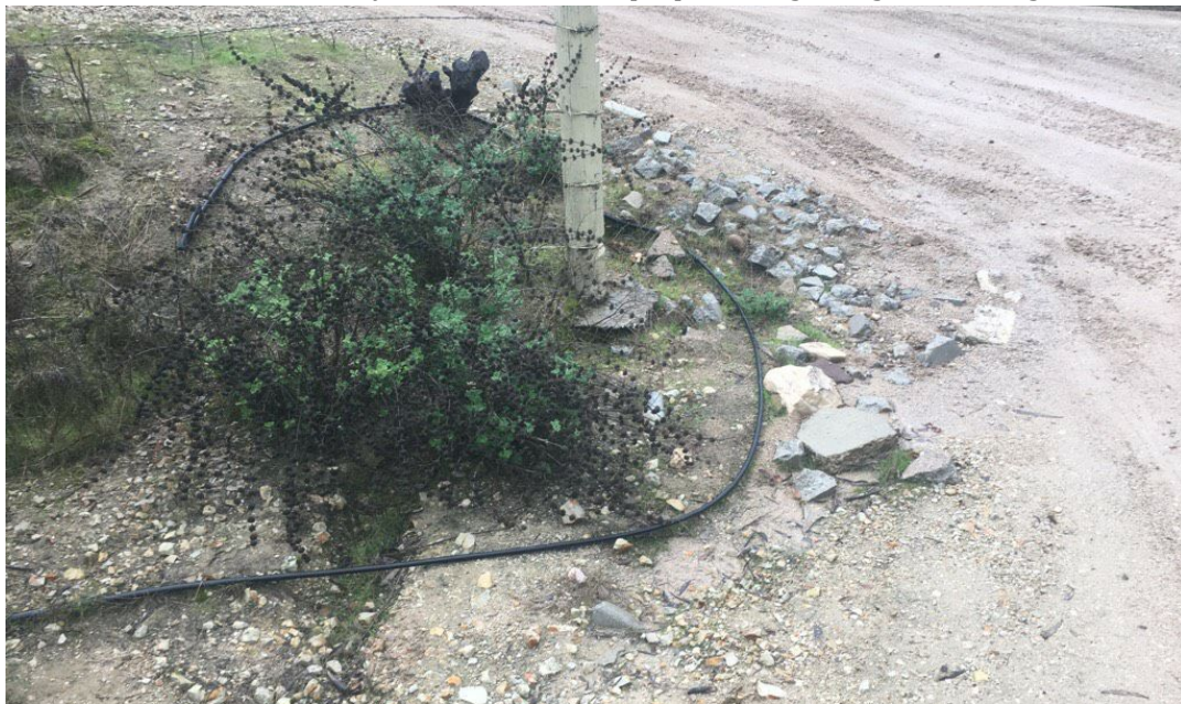
Figure 2-6 Erosion at driveway entrance due to improper road grading and drainage
