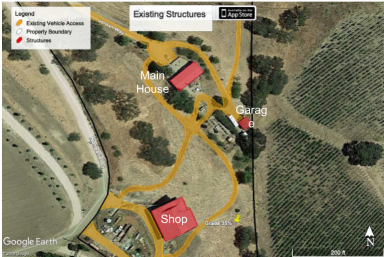
Figure 4-1 Existing structures at Morning Doe Ranch
